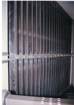
Turning vanes move the airflow around corners.
