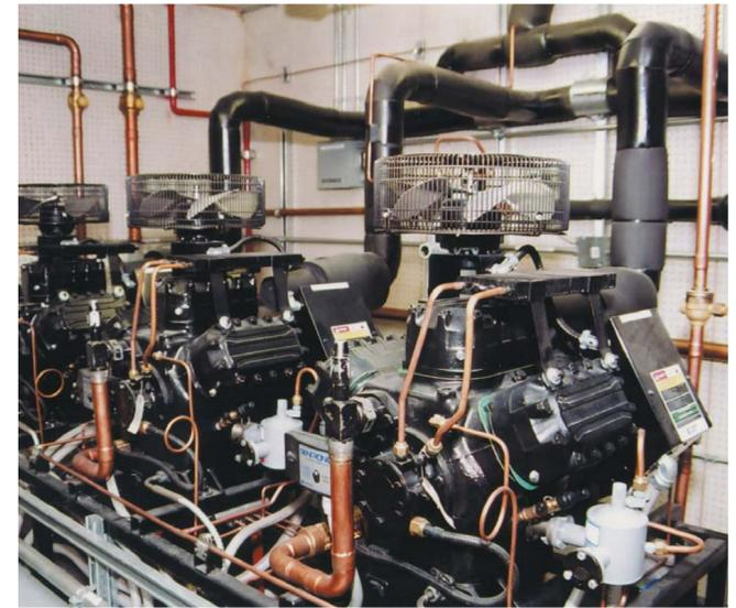
Three 30-hp compressors drop the air temperature to a frigid -37°C.
