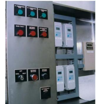
Relay-logic controls make the wind tunnel easy to operate and service.
